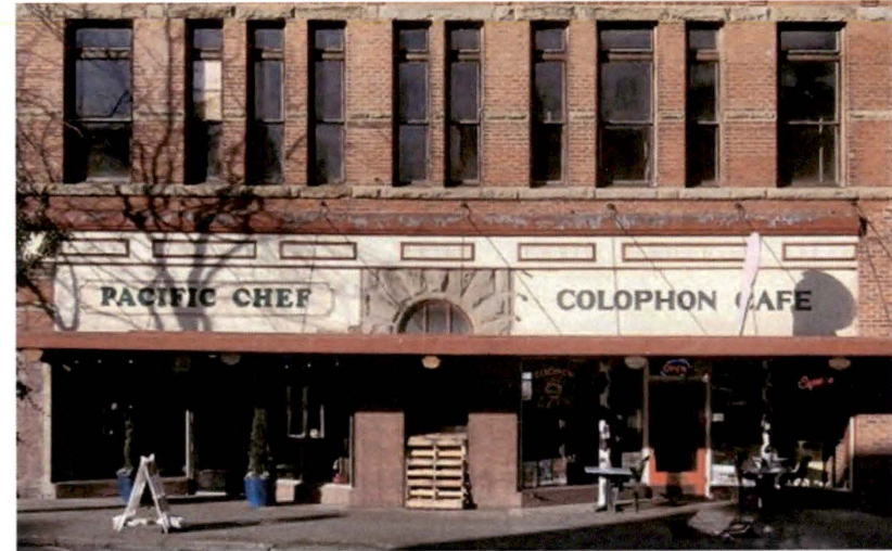
Although obscured with a sign band, the storefront transom windows of the Knights of Pythias building remain intact and could be uncovered and restored in the future.
