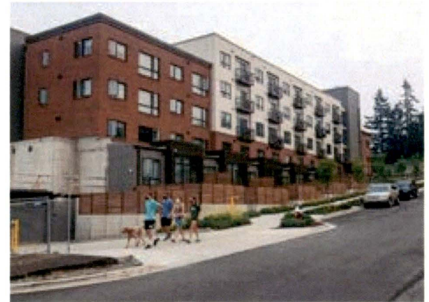
Intersection of N Samish Way and Otis Street, looking southwest on the Samish Commons (1000 Otis St, newly completed affordable housing complex)
