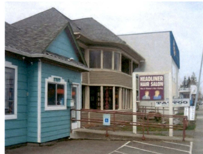
Residential homes converted to commercial purposes adds character to the Fountain District on Meridian Street. As possible, it is recommended that these forms be preserved.
