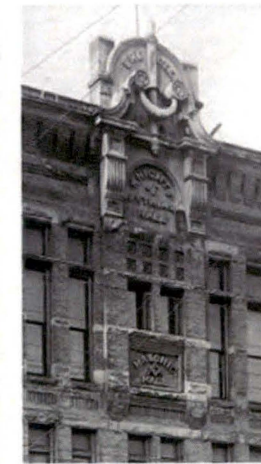
Although portions of the Knights of Pythias building's ornate parapet are missing, the building still presents a powerful presence in the Fairhaven National Historic District. What remains has been preserved and provides a reference to the original design. (Photo at right courtesy Whatcom Museum Photo Archives.)
