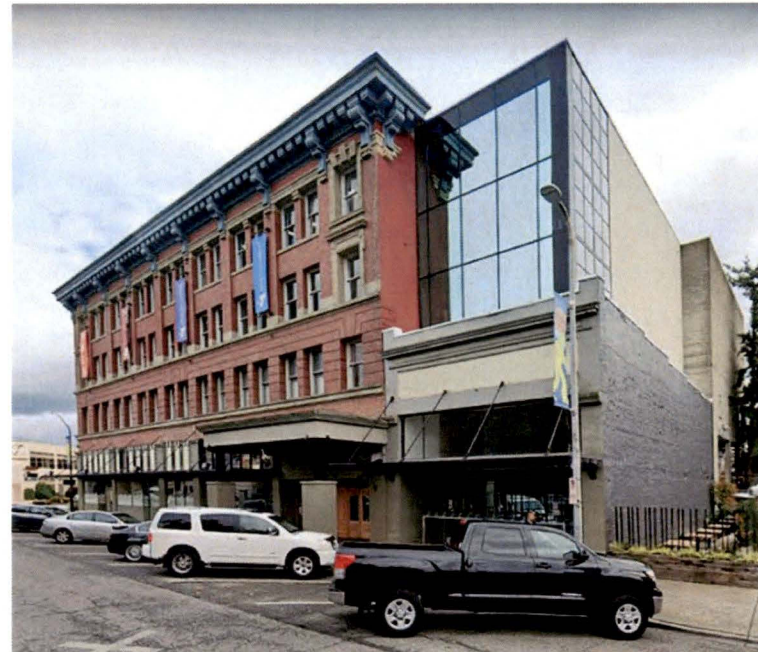
The YMCA was able to expand by purchasing the adjacent one-story building and create a climbing wall by setting-back the roof top addition.
