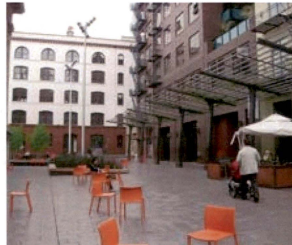
Make plazas wide and flexible enough to accommodate markets and special events.
