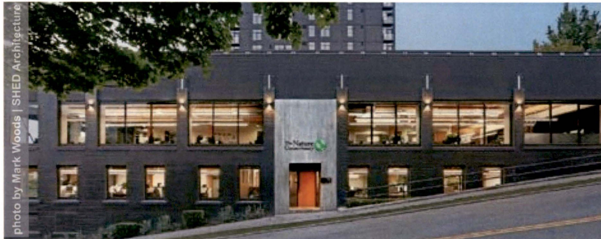
Respect existing historic building features, as well as the surrounding context.
