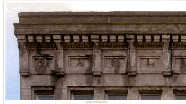
The raised metal letters in the cornice work of the Dahlquist Building, 1311 N. State Street, add character to the building.
